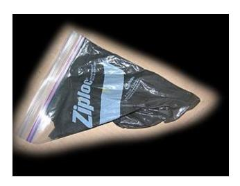
6. Place the mixture in a zip lock bag (shown above), clip the corner of the bag, and squeeze the viscous fluid into the gap (shown below). Keep filling as needed. The mixture will slowly flow throughout the gap, with occasional air bubbles rising to the surface. You may need to add a little more after the first batch has cured and settled.
